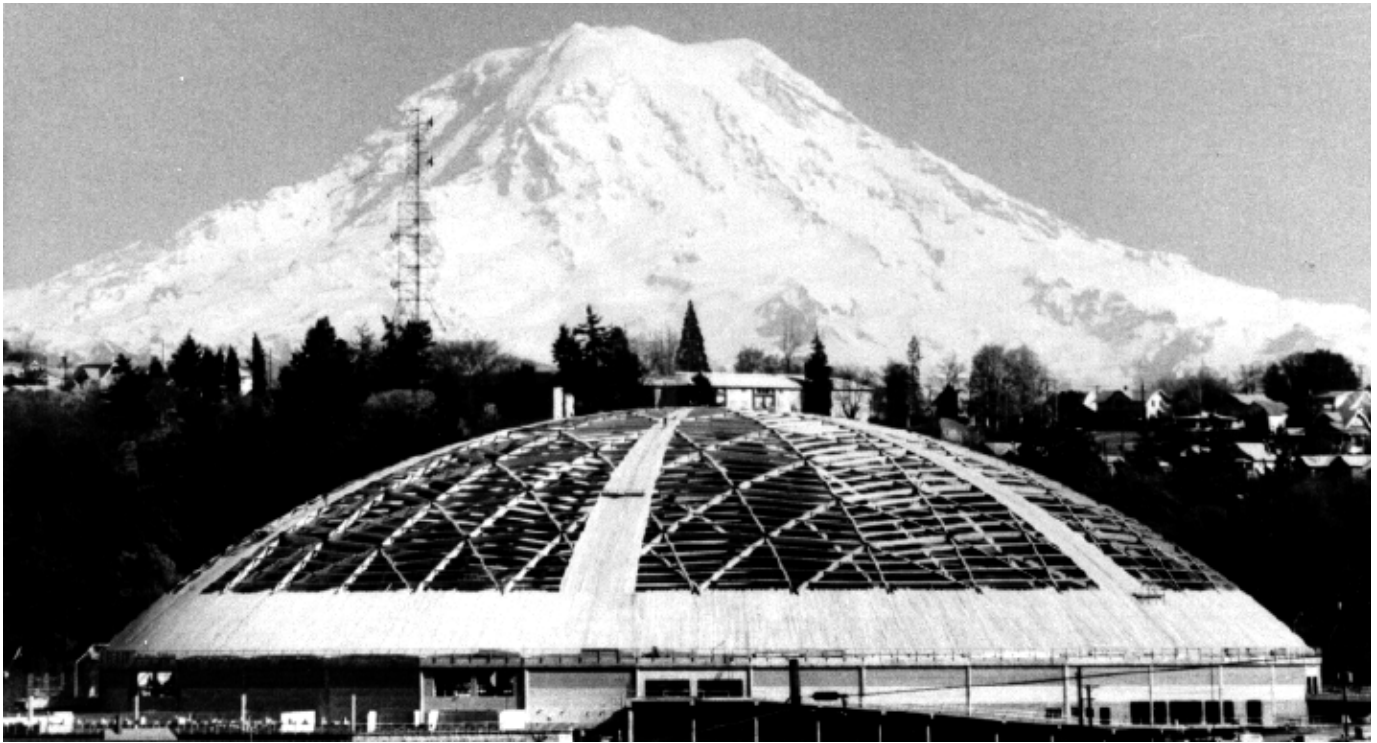
Figure 16–8. This 161.5-m- (530-ft-) diameter Tacoma dome (Tacoma, Washington), built in 1982–1983, is one of the longest clear roof spans in the world. (Photo courtesy of Western Wood Structures, Inc., Tualatin, Oregon.)
