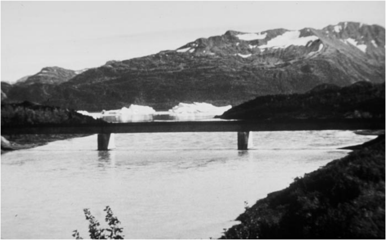
Figure 16–9. Glulam beam bridge over the Dangerous River, near Yukatat, Alaska, consists of three 43.5-m (143-ft) spans. Each span is supported by four 2.3-m- (91.5-in.-) deep glulam beams.
